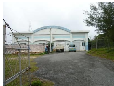
[多良間浄水場]
